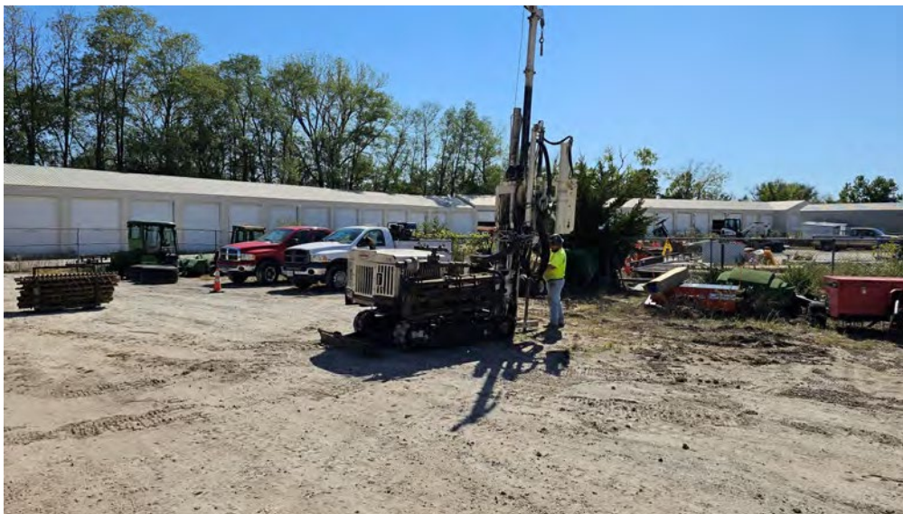
2. Soil Boring SB-3.
