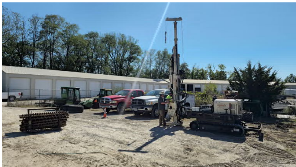
3. Soil Boring SB-4.
