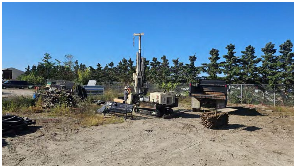
1. Soil Boring SB-1.
